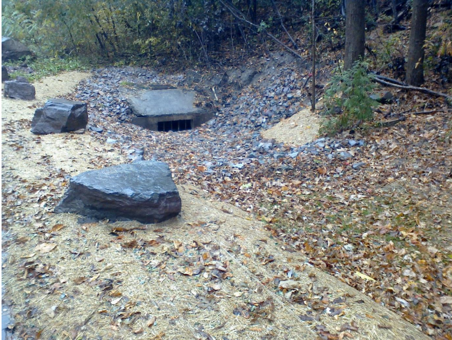
Improved swale along Flynn Ave and surface flow entrance into CB 3
