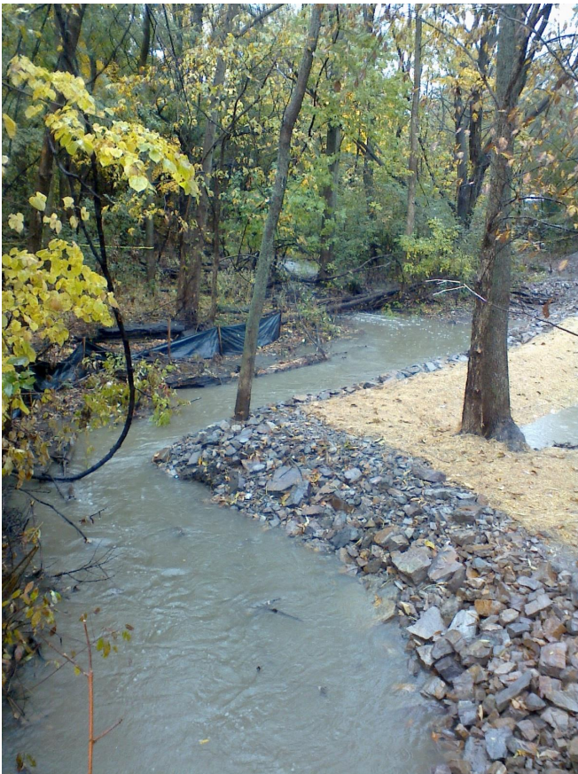
Oakledge Tributary and new berm along new wetland cells
