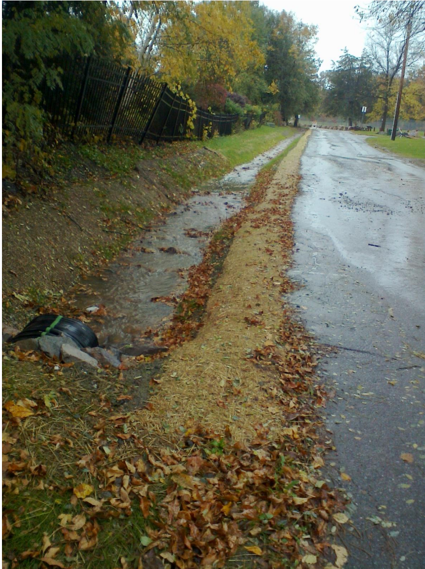
Improved swale during October 19 rain storm
