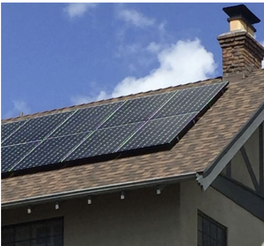
Solar array mounted on an historic home.
