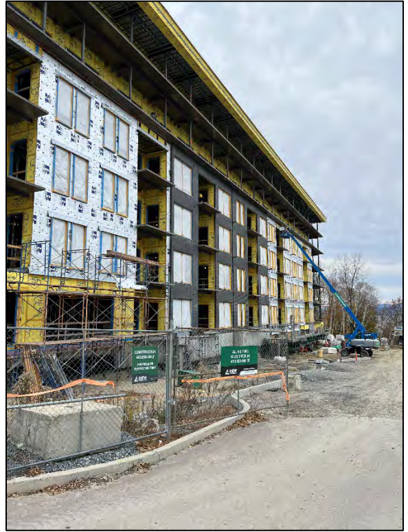
Photo 2: New apartment building south of Lot 8.
