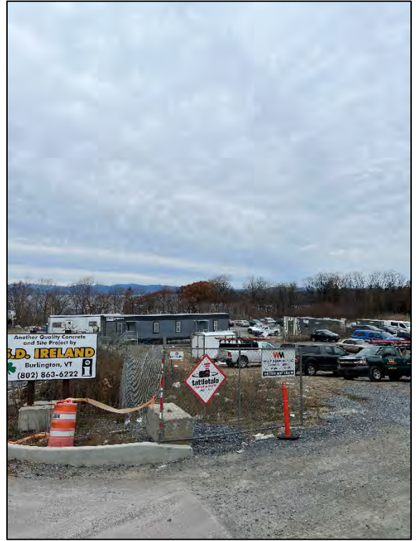
Photo 6: Temporary construction offices.
