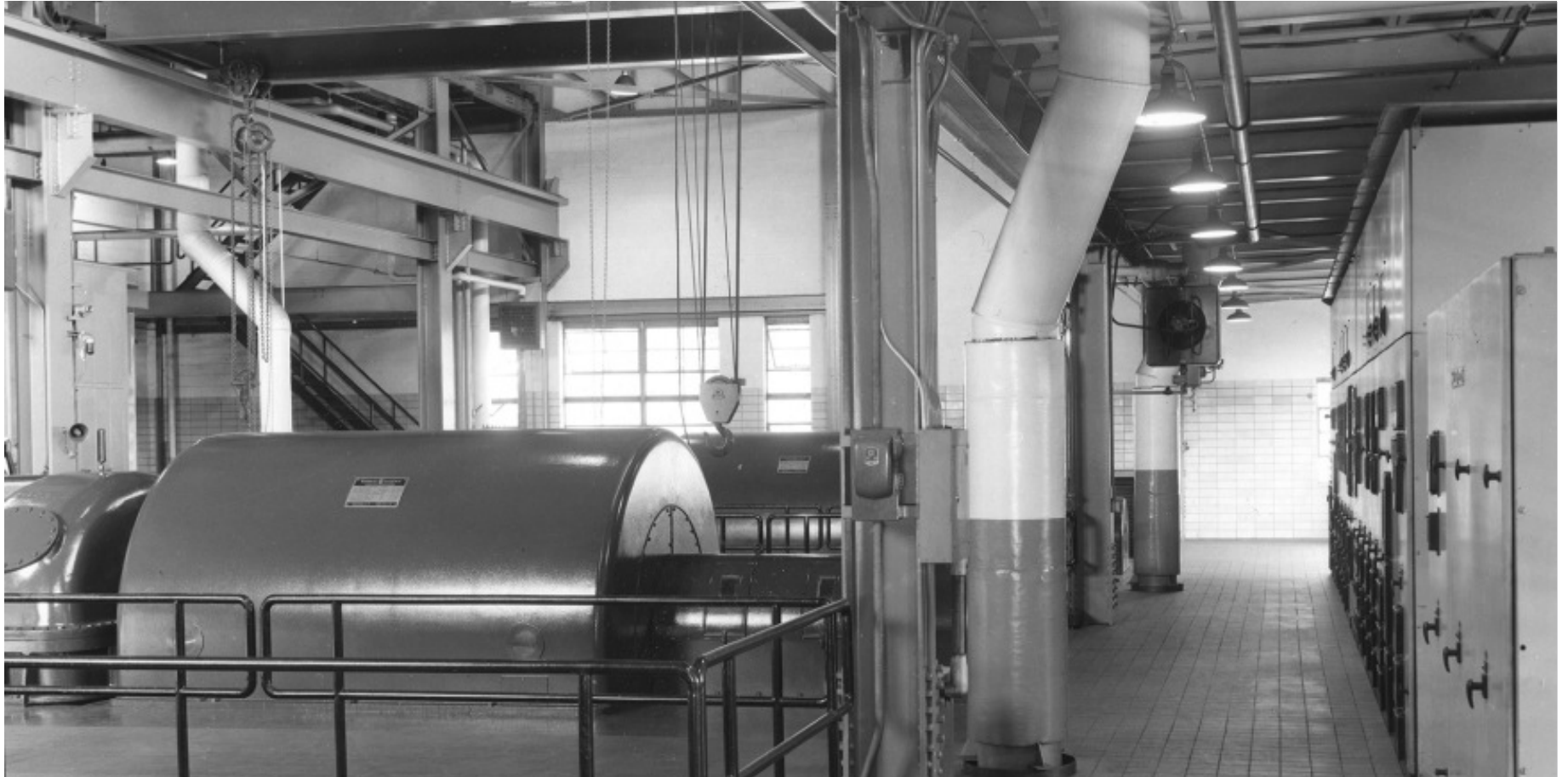
Figure 3.9: Turbine room inside the Moran Plant showing two of the Westinghouse turbines, the unfinished walls, exposed steel beams, and the tile floor. Source: Burlington Electric Department.
