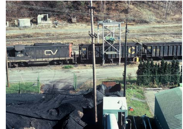
Figure 4.3: 1970s photograph of a train offloading coal at the Moran Plant. Coal was hoisted from the rail car and carried overhead on a wire system to the coal storage yard. Source: Burlington Electric Department.
