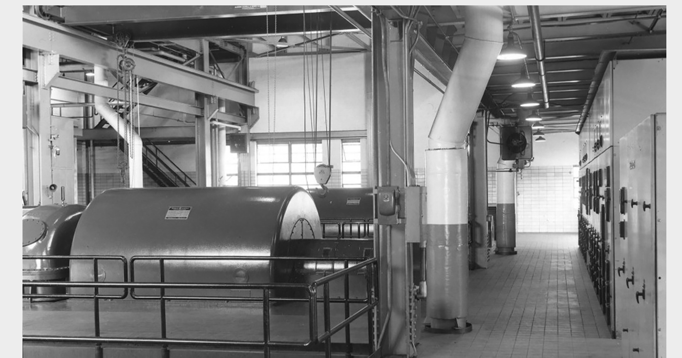
Inside the Turbine Room of the Moran Plant main floor. The turbines are at the center and the switchgear cabinets are to the right. Note the heavy steel frame visible today and the wide, unobstructed walkways surrounding the generating equipment. Source: Burlington Electric Department
