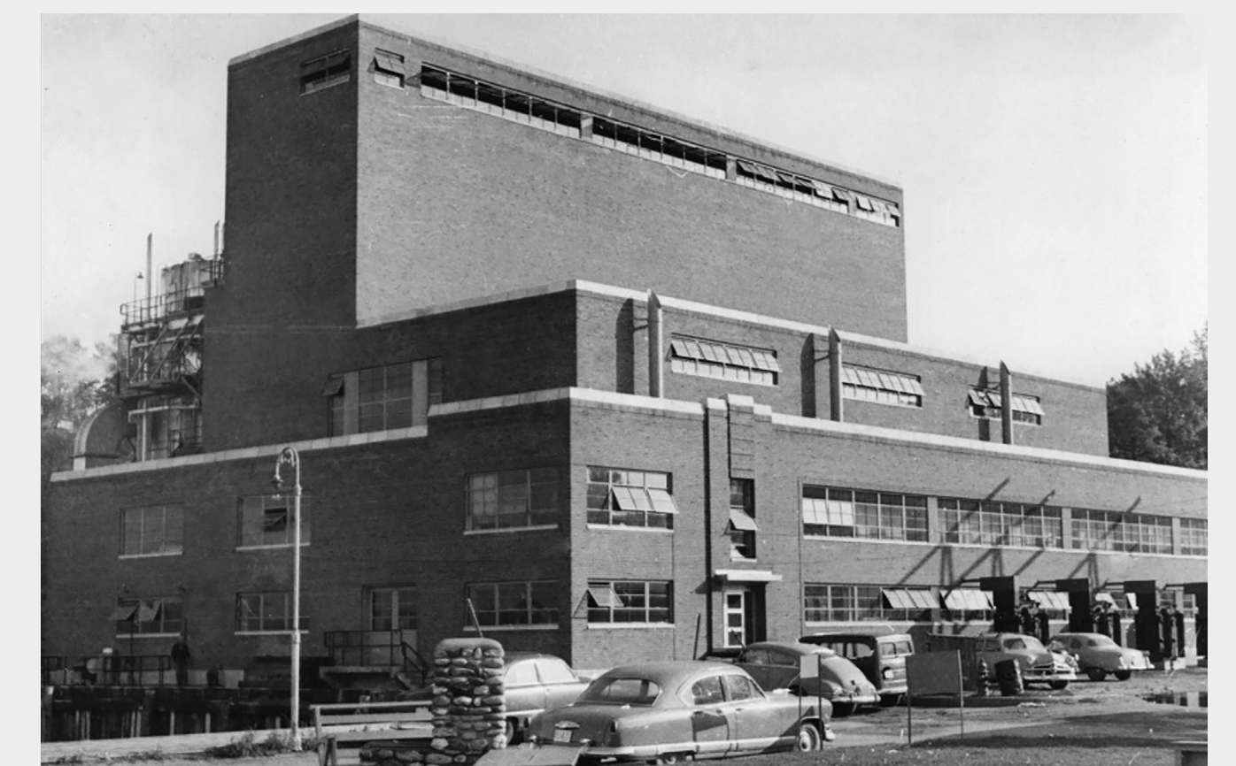
Moran Plant viewed from the southwest. The building's overall form reflected its interior functionality, with the highest portion housing the hoppers that fed coal to the boilers. Source: Burlington Electric Department
