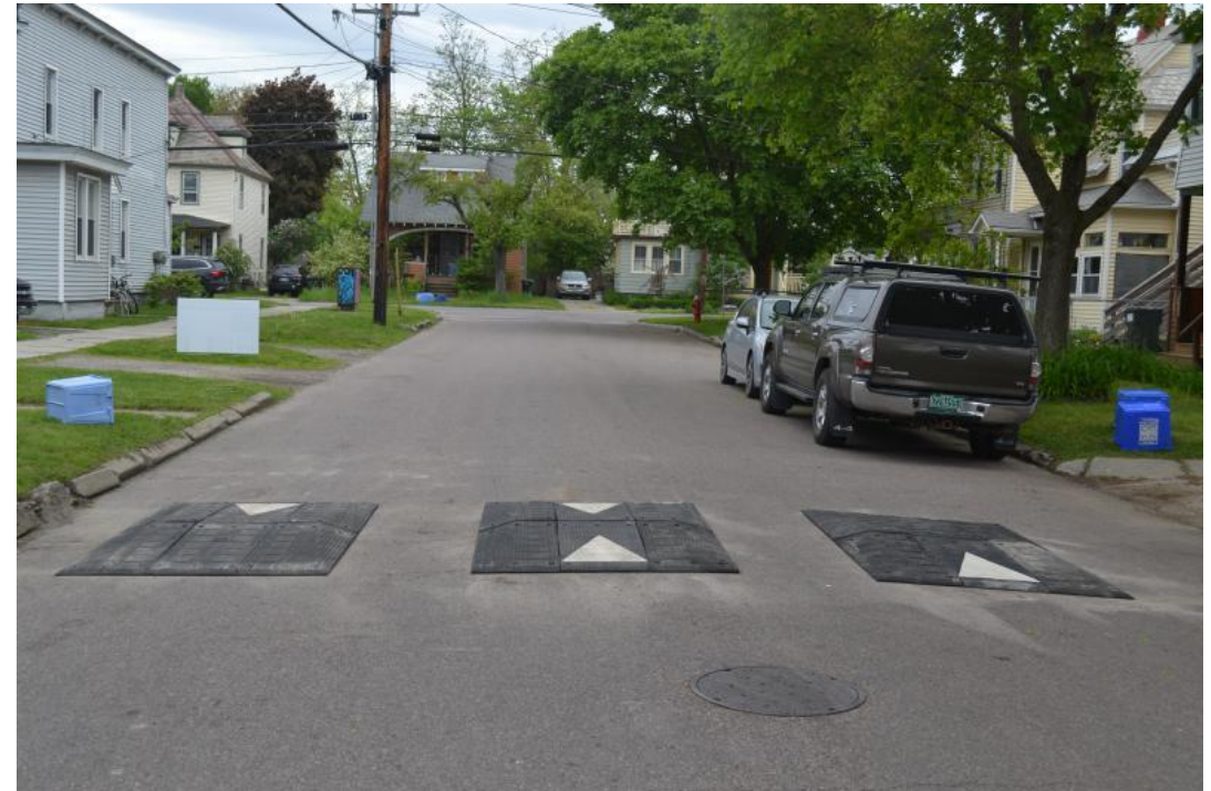
Ward Street Traffic Calming using speed cushions
