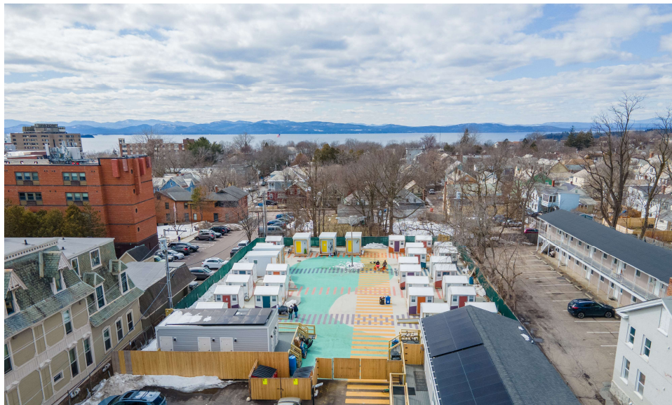
Aerial Image of Elmwood Community Emergency Shelter
