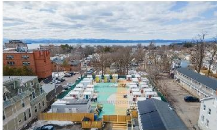
Aerial Image of Elmwood Community Emergency Shelter
