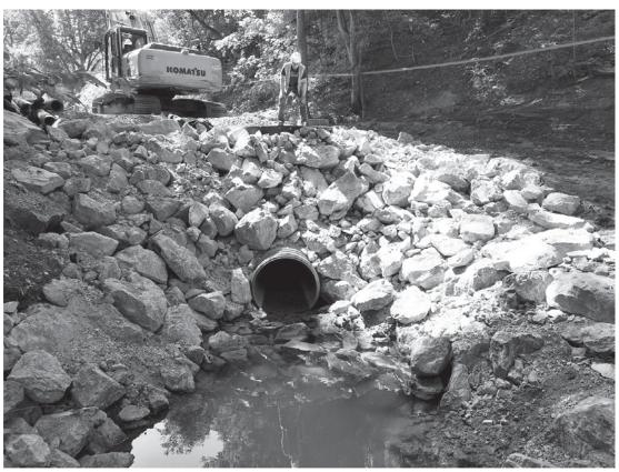
Completion of the Gazo outfall repair project. This is the end of the new outfall pipe
