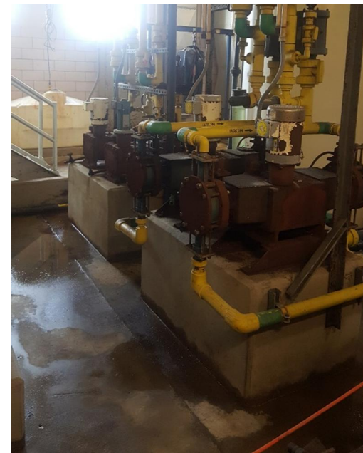
Bromine pumps: 24 years old; critical to disinfection of wet weather
