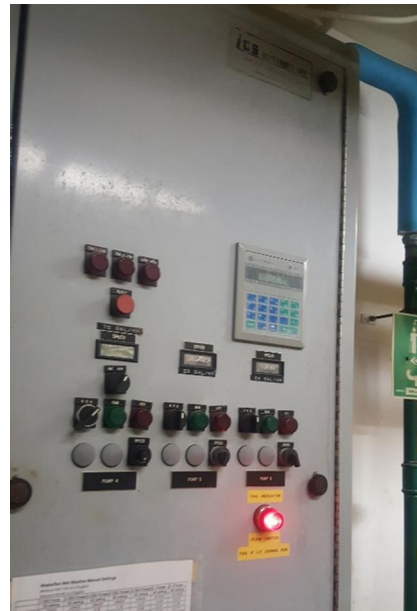
Disinfection system control panel: only one switch (hand-off-auto) works. Other control panels have obsolete parts that cannot obtain anymore..
