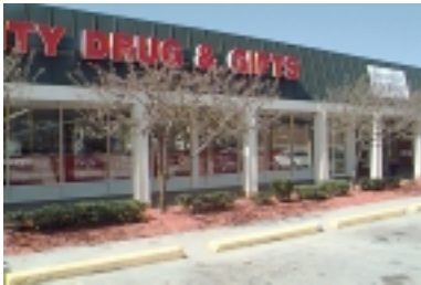
Landscaping in a commercial facelift
