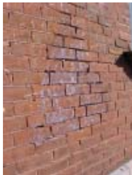
Mortar damage
