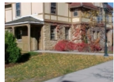
An extension to the sidewalk has been created linking the porch and walkway with a smooth and gradual route.
