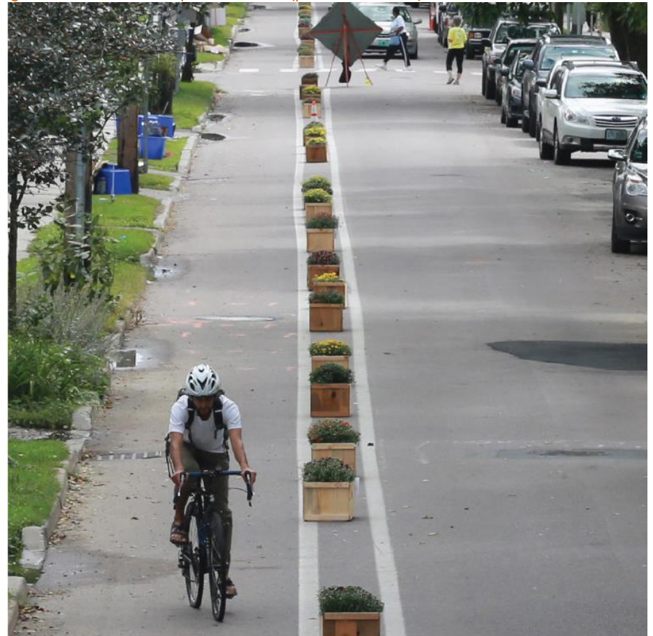
Figure 4.15: Planted Buffer pilot installation (planBTV Walk Bike)
