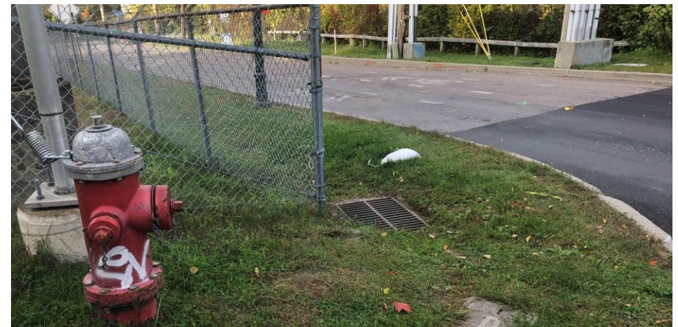
Drainage / Utility Relocation and Improvements
