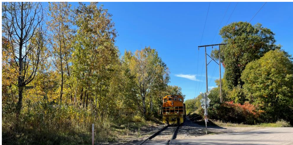
Railroad Crossing Safety Improvements
