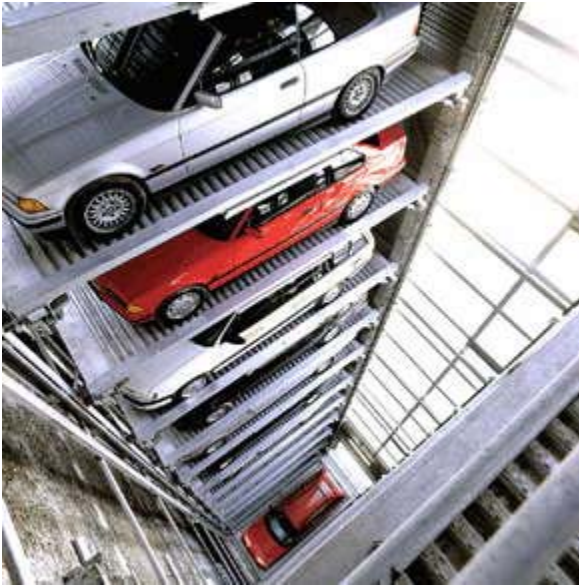
Figure 8: Interior of Automated Parking System (source: SpaceSaver Parking Systems)
