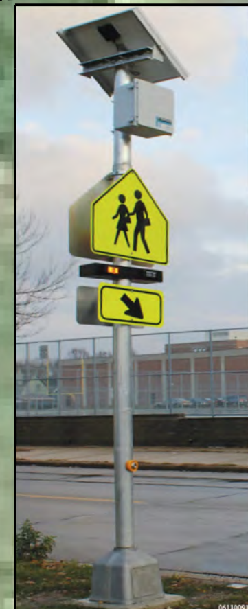
PEDESTRIAN ACTUATED W/SCHOOL CROSSING, (2) S1-1 W/RECTANGULAR RAPID FLASHING BECON (RRFB)
