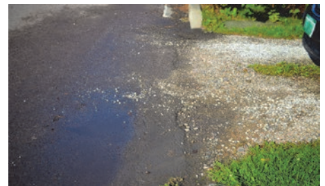
A Burlington gravel driveway without proper slope and drainage. Gravel and oils are washing into the street.
