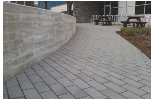
A concrete paver walkway in Burlington.
