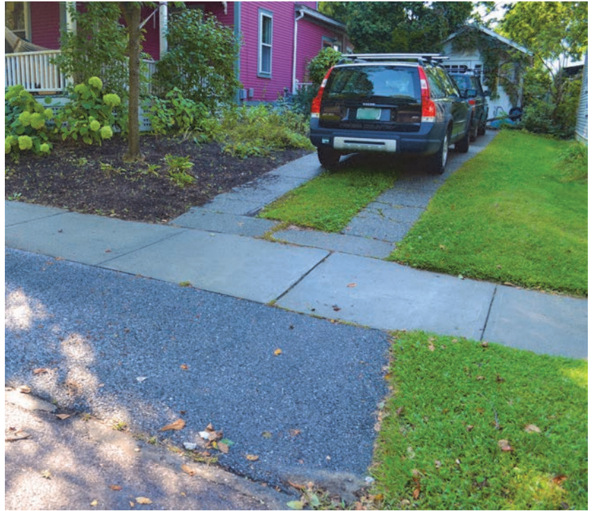
A ribbon or "Hollywood" driveway, like this one in Burlington, is another stormwater-friendly driveway option.
