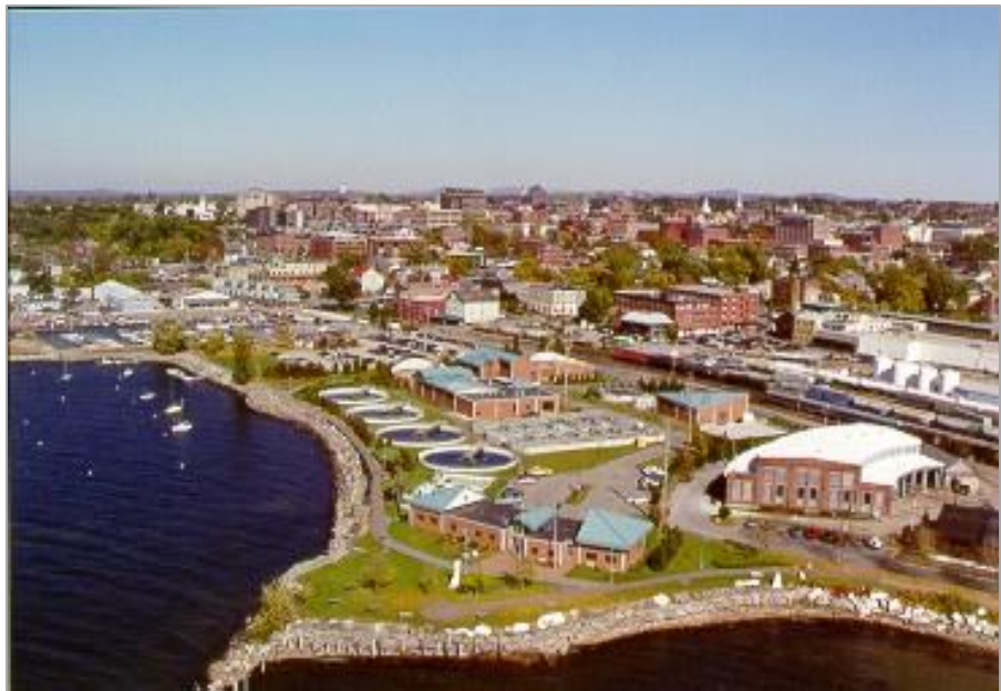
Burlington Main WWTP located on Burlington’s waterfront
