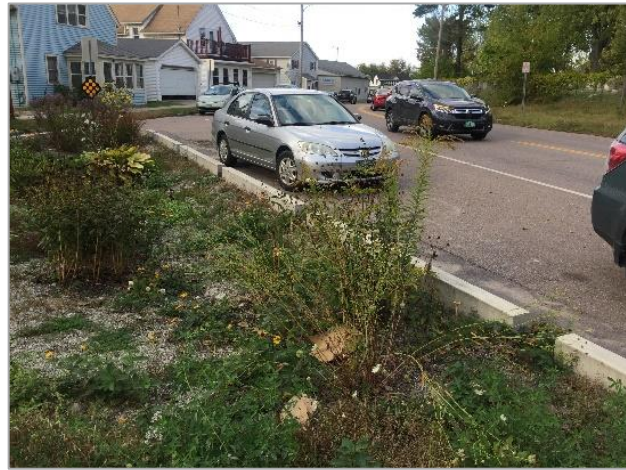
Infiltration Stormwater Treatment Practice on North Willard Street, 2010
