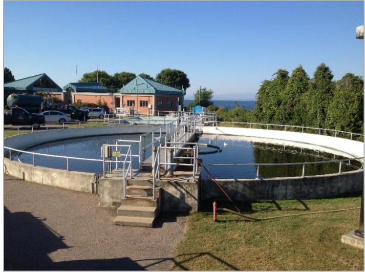
Secondary clarifier at Burlington Main WWTP
