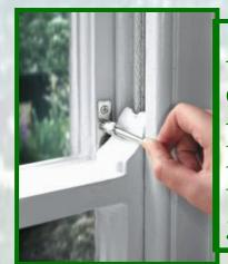
A variety of keyed window locks for both the corner and the sash are available at common hardware stores, and serve the same function as the key-only deadbolt on the door. Even if the window glass is broken, the window is still secured.
