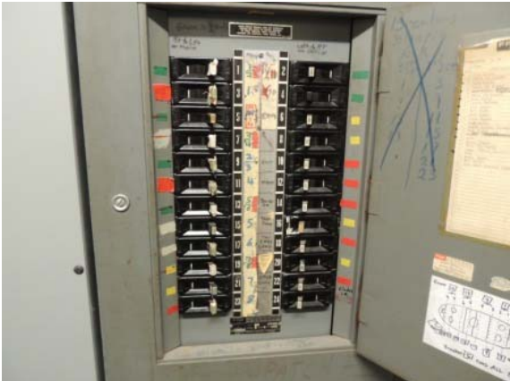
Photo #7: Original Federal Pacific Secondary Panel (typical throughout the building) in Need of Replacement
