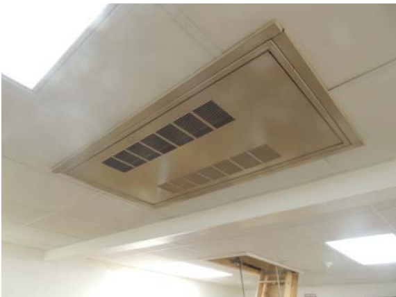
Photo #36: Typical Ceiling Mounted Hydronic Hot Water Heater
