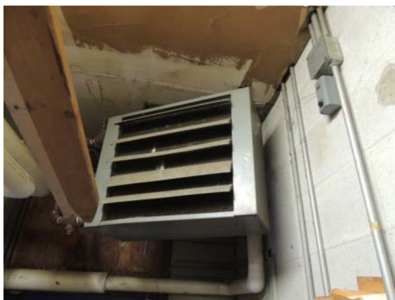
Photo #16: Hydronic Unit Heater located in the Main Mechanical Room
