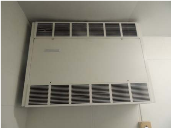
Photo #37: Typical Wall Mounted Hydronic Hot Water Heater
