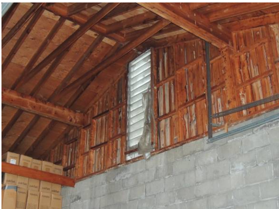
Photo #60: Building Ventilation Louver Serving the Maintenance Building
