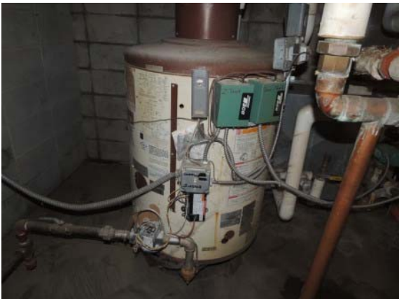
Photo #11: A.O. Smith Domestic Hot Water Boiler located in the Main Mechanical Room
