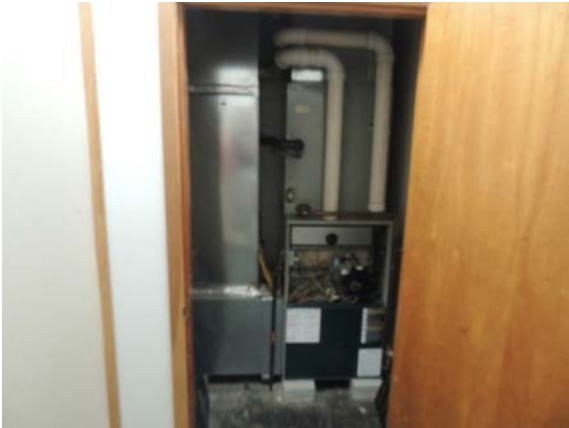
Photo #31: American Standard Gas-Fired Furnace with Cooling Coil supplying the Main Office Area located on the Second Floor
