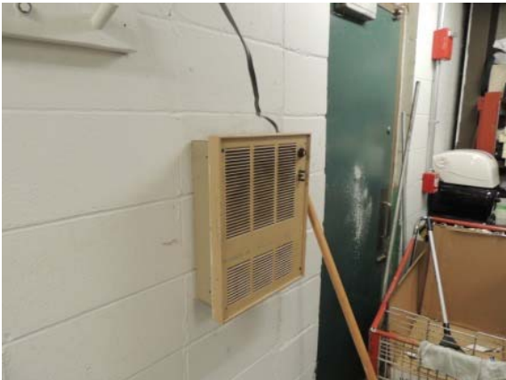
Photo #39: Typical Wall Mounted Electric Unit Heater
