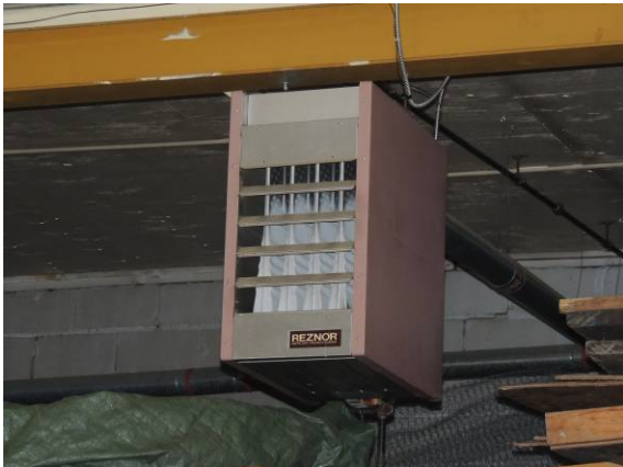
Photo #58: Gas-Fired Unit Heater Serving the Maintenance Building (typical)
