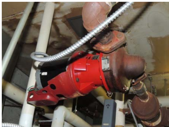
Photo #13: Bell & Gossett Circulation Pump located in the Main Mechanical Room
