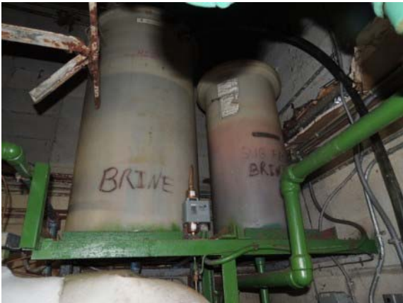
Photo #22: Brine Tanks for the Ice Making Equipment which Leak
