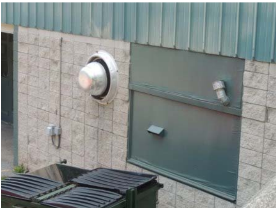
Photo #47: Typical Side Wall Building Exhaust Fan
