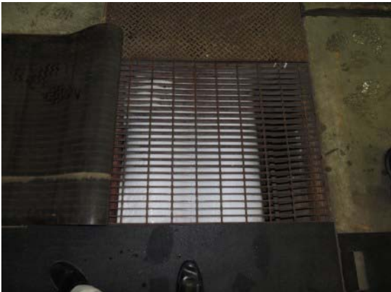
Photo #24: Ice Build-Up on Ice Making Supply Piping located in a Floor Trench
