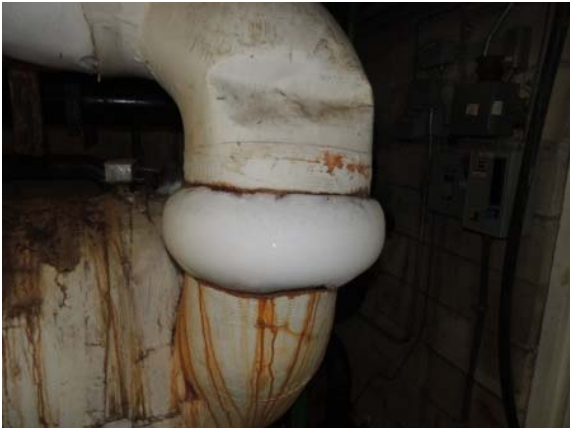
Photo #20: Ice Build-up on the Ice Making Equipment Piping
