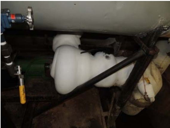
Photo #21: Ice Build-up on the Ice Making Equipment Pump
