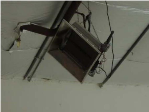
Photo #29: Typical Modine Gas-Fired Radiant Heaters located above the Main Grandstand
