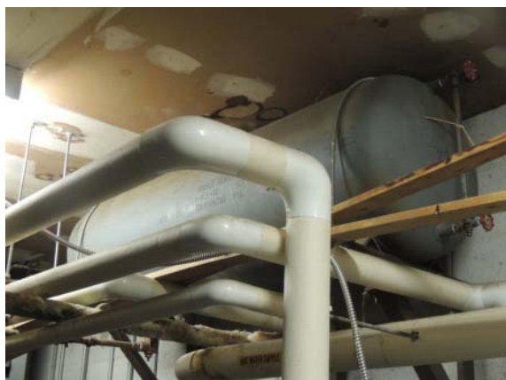
Photo #15: Expansion Tank located in the Main Mechanical Room
