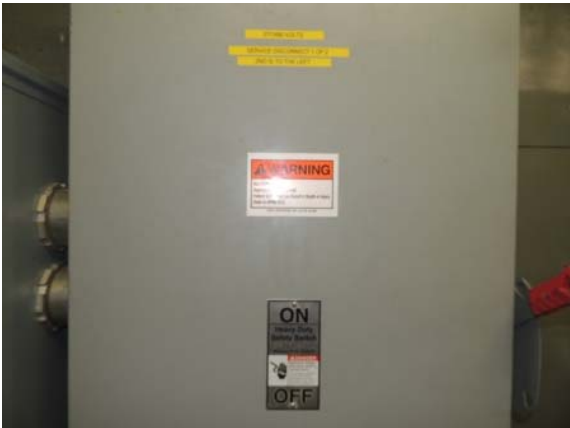
Photo #6: New Square D Incoming Electrical Service Panels replaced in 2014
