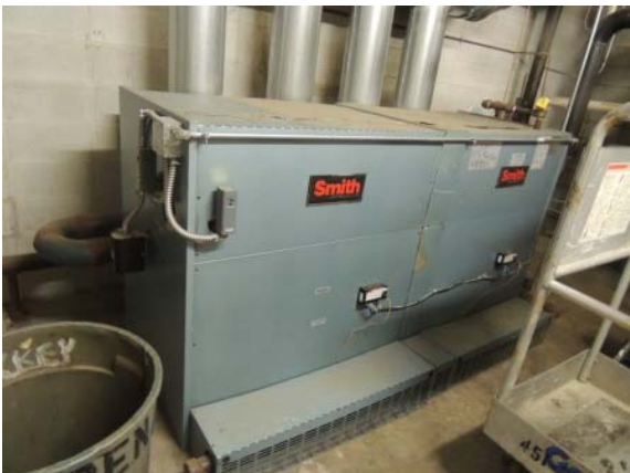
Photo #10: Smith Gas-Fired Heating Hot Water Boilers located in the Main Mechanical Room
