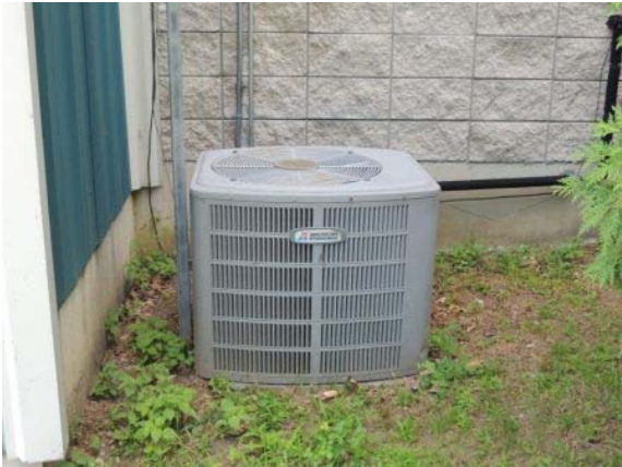
Photo #32: American Standard Air-Cooled Condensing Unit supplying the Main Office Area located on the Second Floor
