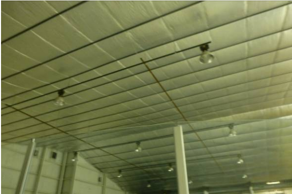
Photo #50: Ceiling insulation
