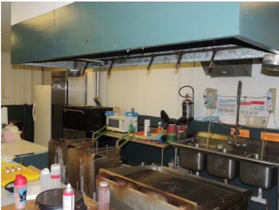
Photo #40: Concession Kitchen Exhaust Hood with Ansul Fire Protection
