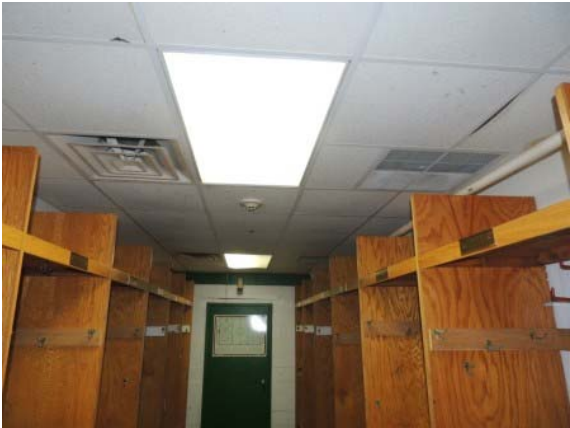
Photo #49: Typical Locker Room Recessed Florescent Lighting
