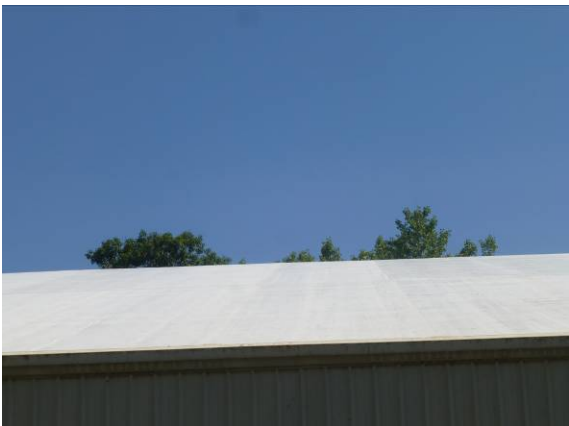
Photo #23: TPO roofing
