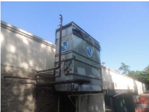
Photo #33: Baltimore Air Coil Cooling Tower supplying the Ice Making Equipment located at the West Elevation
