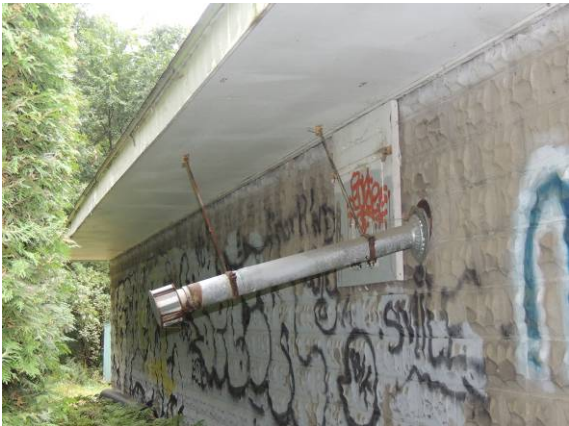
Photo #57: Unit Heater Exhaust Flue Serving the Maintenance Building (typical)
