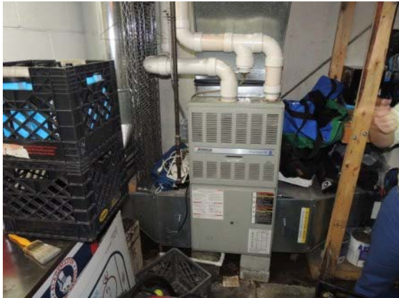
Photo #30: American Standard Gas-Fired Furnace (No Cooling) supplying the High School Locker Rooms located below the Main Grandstand
