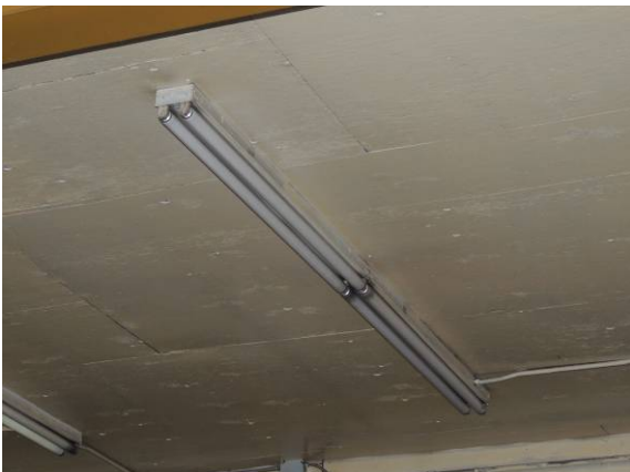
Photo #59: Surface Mounted Florescent Lighting Serving the Maintenance Building (typical)
