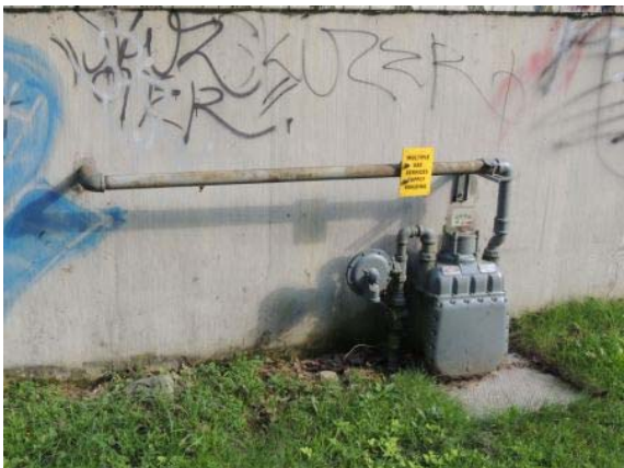
Photo #2: Secondary Natural Gas Meter at North Elevation of Building
