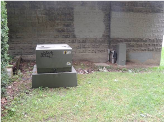
Photo #55: Electrical Transformer Serving the Maintenance Building
