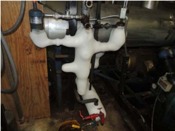
Photo #19: Ice Build-up on the Ice Making Equipment
