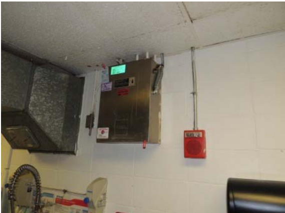
Photo #41: Concession Kitchen Ansul Fire Protection Control Panel
