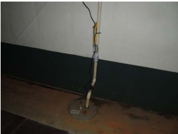
Photo #35: Sump Pump Located under the Main Grandstand
