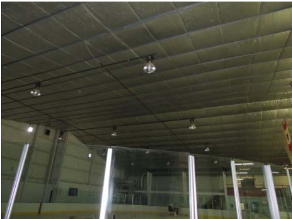
Photo #51: Secondary Rink Metal Halide Overhead Lighting
