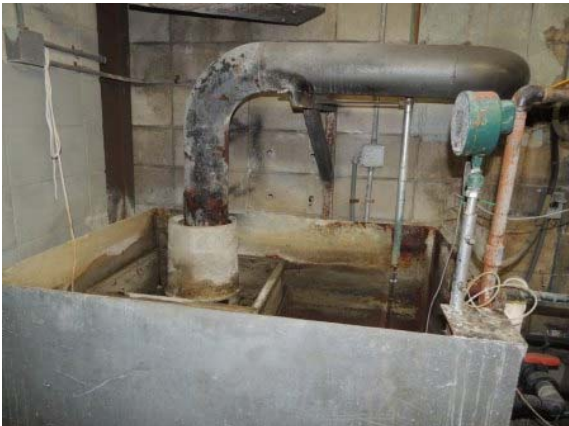
Photo #23: Ice Making Equipment Sump which is Severely Corroded
