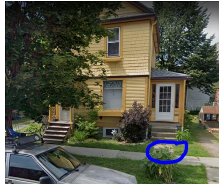
Walkway to be removed
