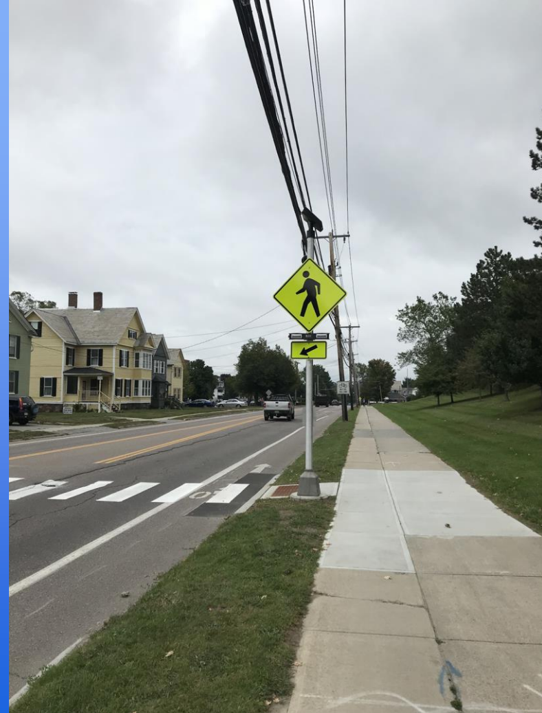
FLETCHER PLACE CROSSWALK W/ RRFB 2018
