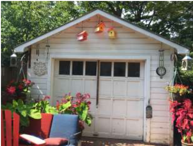
Garage door with wooden rod to keep closed.
