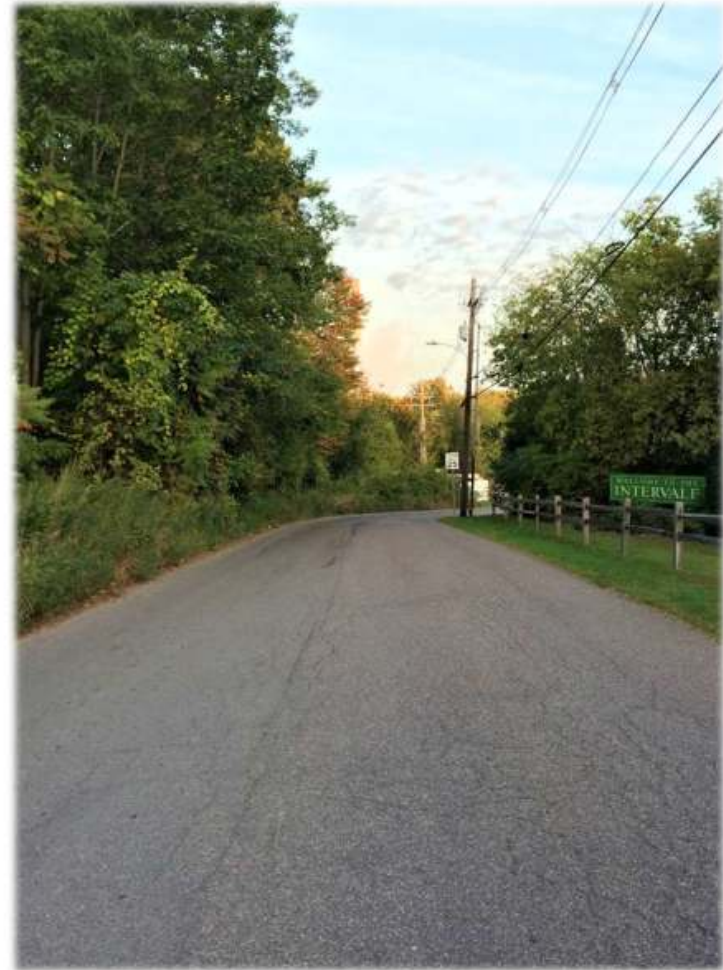
Figure 3: Intervale Road (Looking North from Railroad Tracks)
