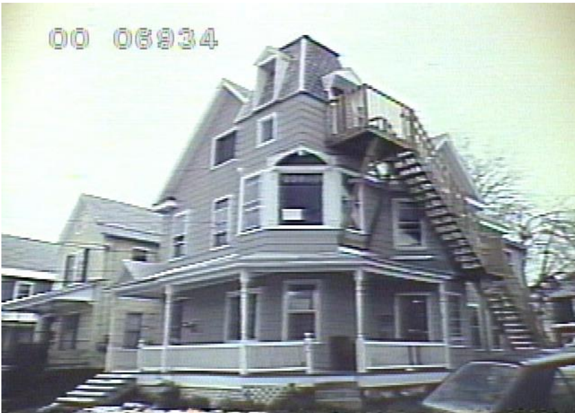
1984-85 Assessor Revaluation photograph Stairs are new build
