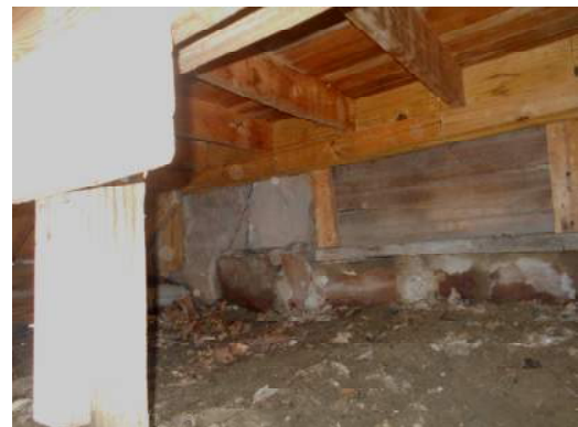
The south wall has several jogs that help stabilize the wall and therefore it does not appear to be leaning inward. The mortar joints are in poor condition with loose stones and missing mortar.
