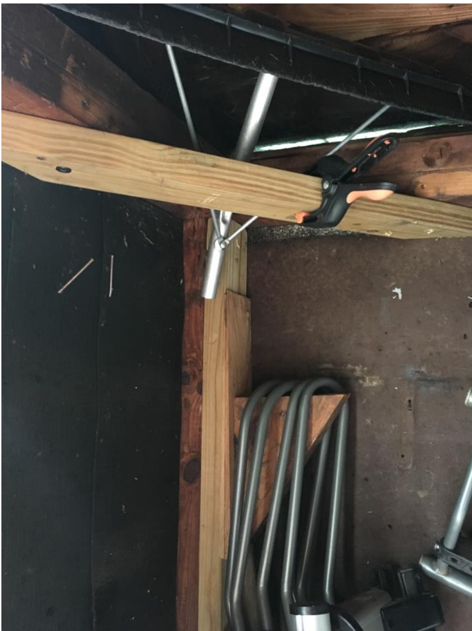
Reinforced corners in fall 2017
