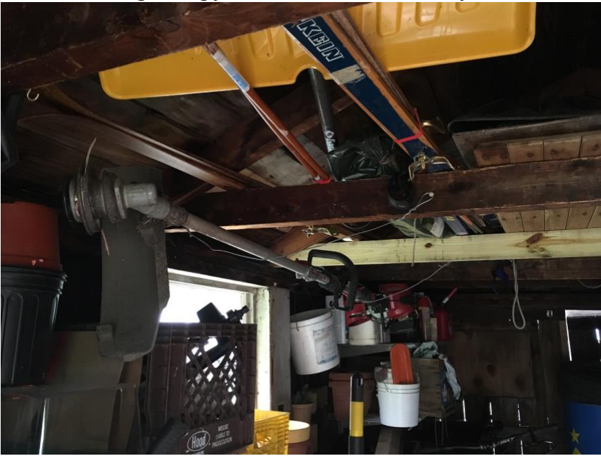
Secured existing ceiling joists and added additional joists in fall 2017
