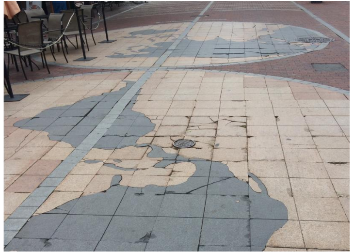
Figure 4: Stone Globe Paver Damage
