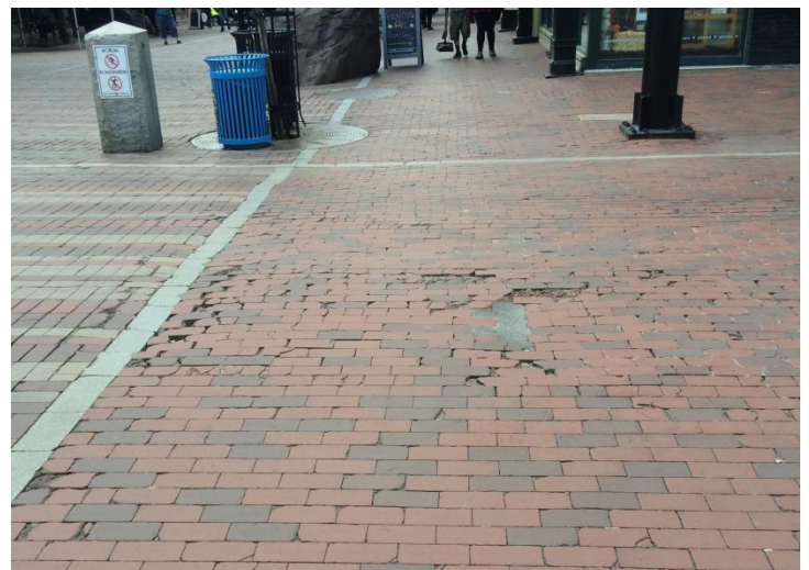
Figure 2: Paver Damage at Bank & Church Streets
