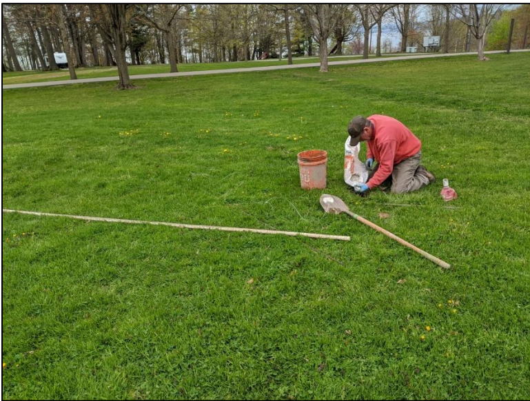
Photo #3: PVC pulled in one piece (or, unscrewed in 10 ft sections at MW-2R).
