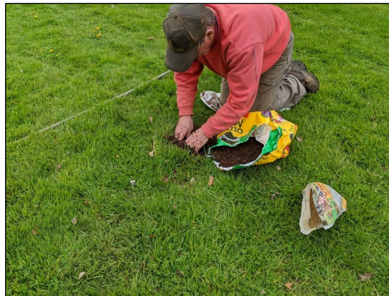
Photo #6: Finishing abandoned well with clean topsoil and grass seed.
