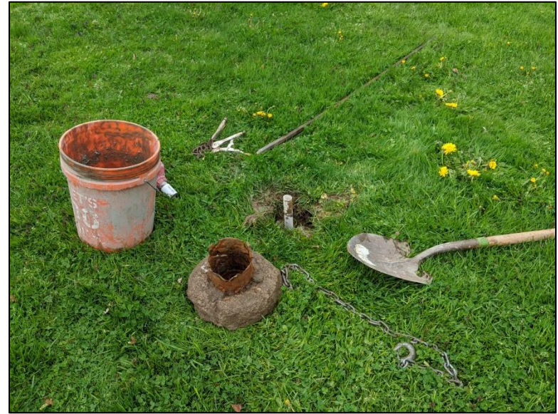
Photo #2: Exposed well, decommissioning tools.
