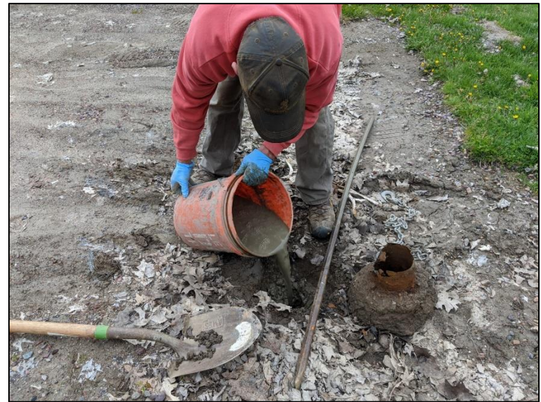
Photo #4: Grouting annular space with bentonite slurry..
