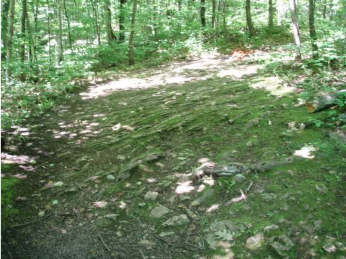
X-Country Course: Tread creep on a wide section of exposed ledge, crushed stone surfacing with retaining rock cribbing are proposed
