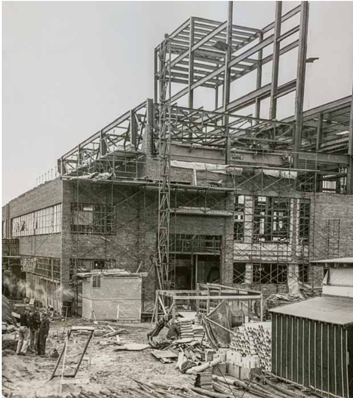
Figure 3.6: The Moran Plant mid-construction in 1954. Note the portion of the exposed steel frame. Source: Burlington Electric Department.
