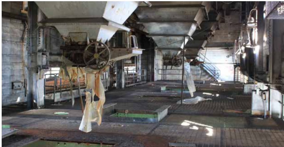
Figure 5. 9: Interior of the Moran Plant showing the coal hoppers. Source: Kaitlin O'Shea, VHB.
