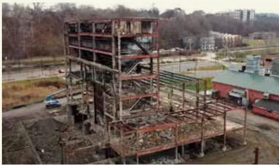
Figure 6.2: The Moran Plant after the brick envelope was removed and during soil restoration efforts. Source: Jeffords Steel and Engineering Company.
