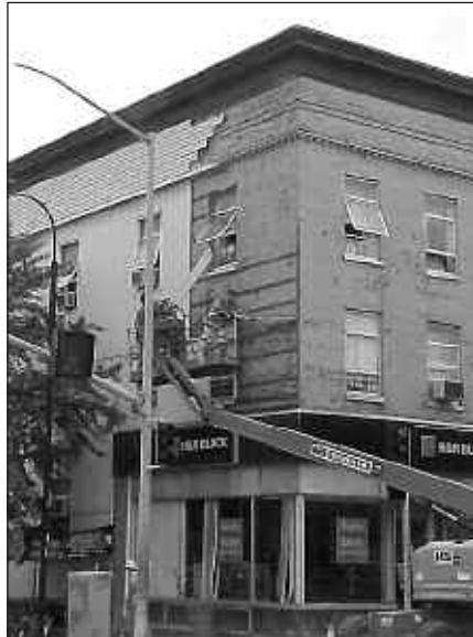
Work performed at 207-217 College Street.
