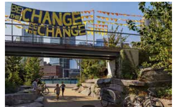
Pedestrian Bridges Connect Park Levels
