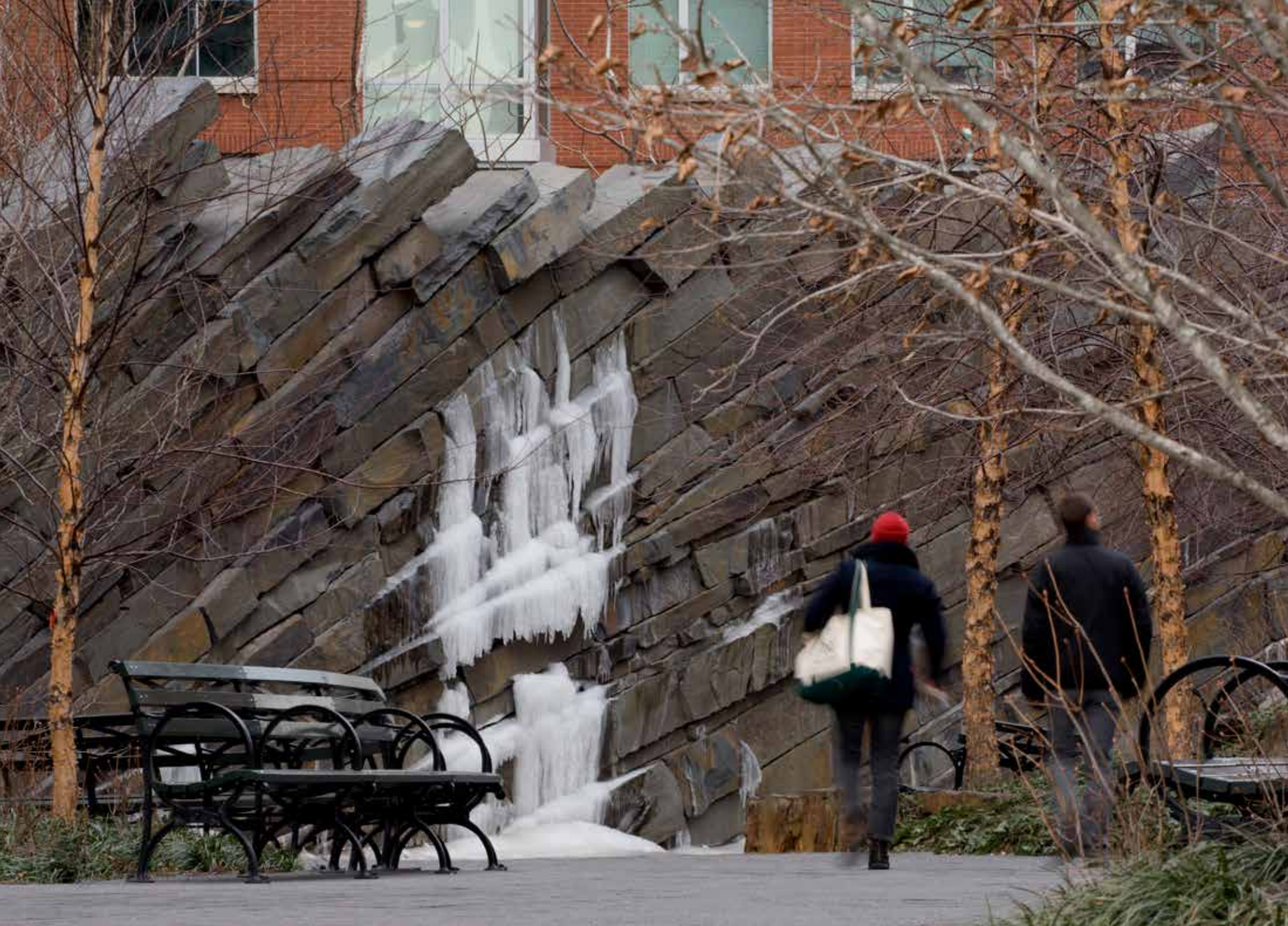
Ice Wall Screens Park Storage & Infrastructure Teardrop Park, New York, NY
