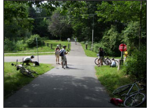
Existing path stop control and limited sight lines to the west at North Avenue Extension
