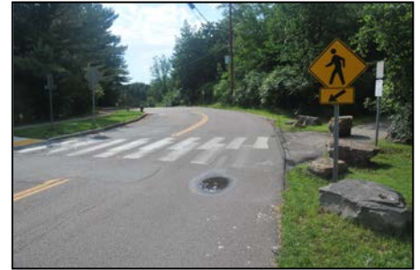
Austin Drive bike path connection showing unmarked boulder and limited sight distance
