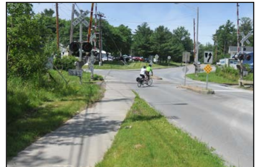
Tandem cyclists unsafely crossing the railroad tracks at a skewed angle
