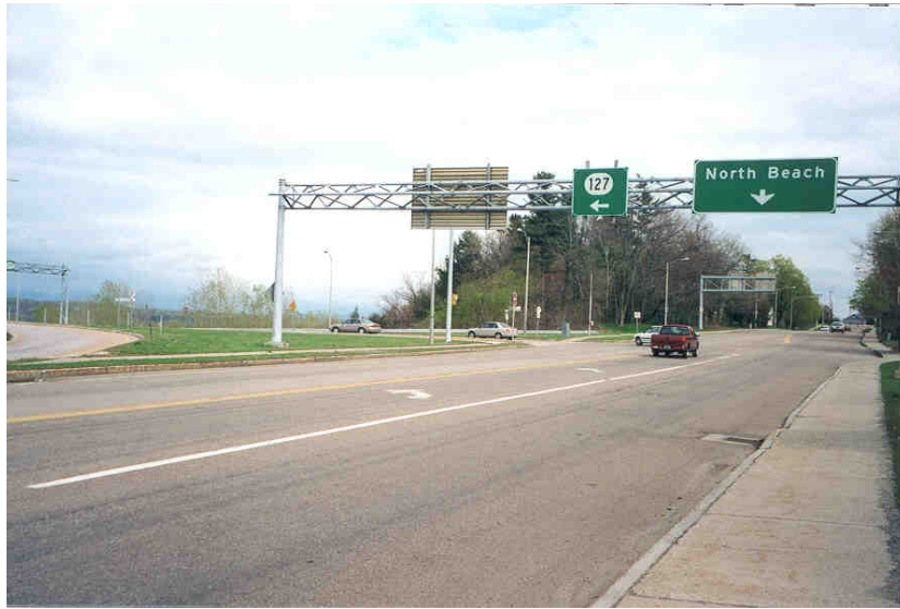
Photograph 3: Looking southbound at the existing North Avenue / Route 127 Intersection (shown here before the traffic signal was added). Note the non-traditional wide lanes, a slip ramp that is designed for high speeds, and an inadequate network for bicycles and pedestrians.
