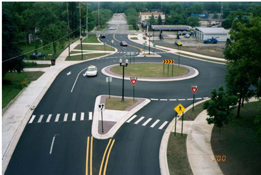
Photograph 7: A one and two lane roundabout in Okemos, Michigan. This design is similar to Alternative E proposed here.
