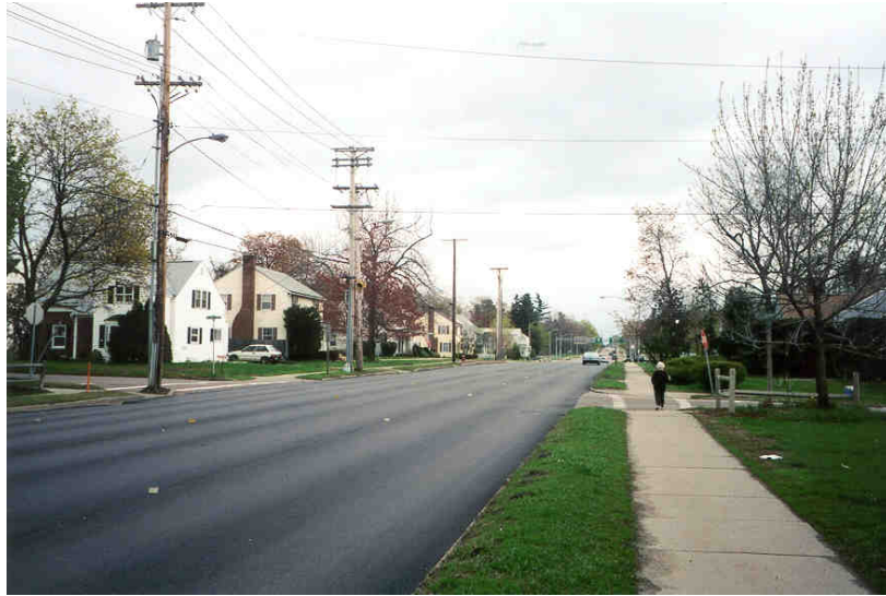
Photograph 4: This photograph, taken looking south on North Avenue from Ethan Allen Parkway, has a green space between the sidewalk and the street for snow storage. The driveways along this corridor sometimes add to conflicts and congestion.
