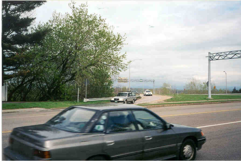
Photograph 5: This photo shows the edge of guardrail adjacent to the north exiting slip ramp off Route 127 where there is a marked pedestrian crossing with limited sight distance..
