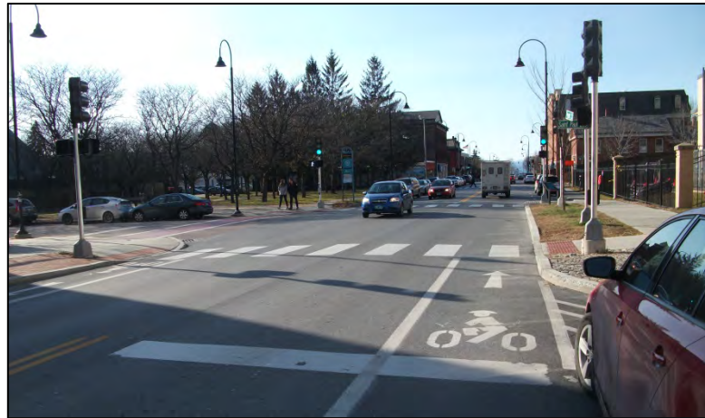
Newly Installed Bike Lane and Curb Extension at St. Paul Street
