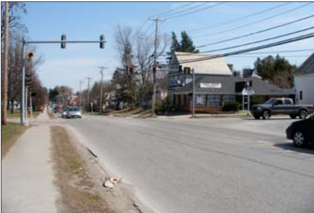
31. Due to a lack of curbing, this narrow green strip receives a lot of vehicular damage.
