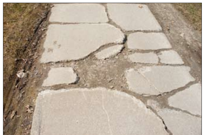
30. Detail of sidewalk damage.
