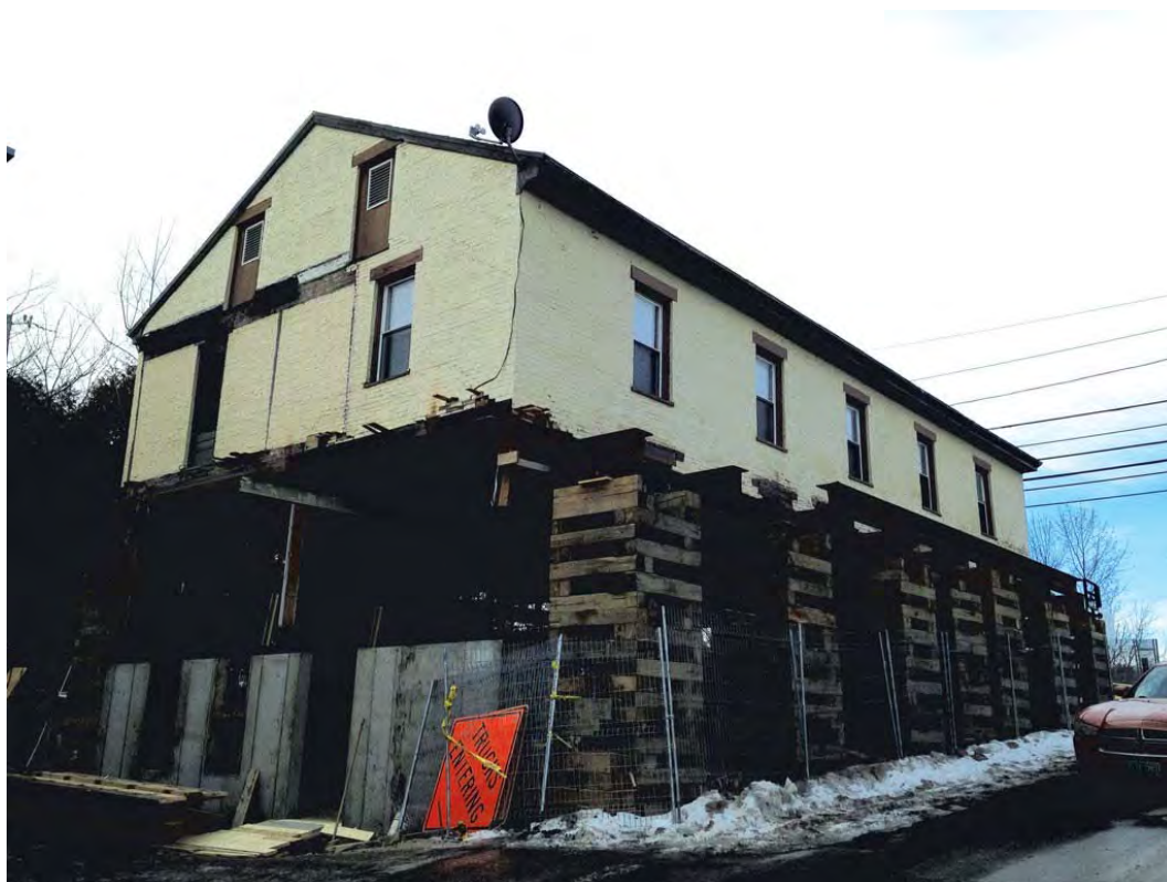
Figure 34. Lifting the second floor of 495-97 Colchester Avenue, c. 2015. View looking southwest.
