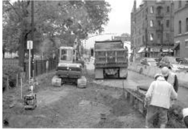
Building new sidewalk on Pearl Street
