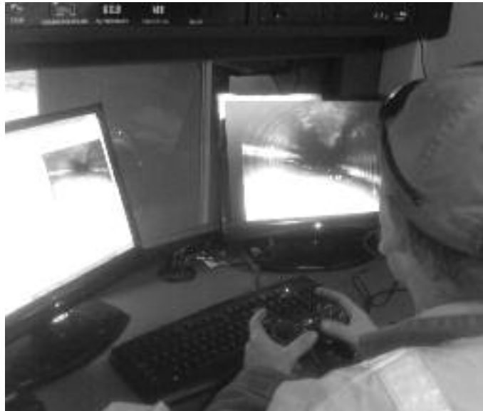
Video inspection of stormwater pipes to determine location of cracks
