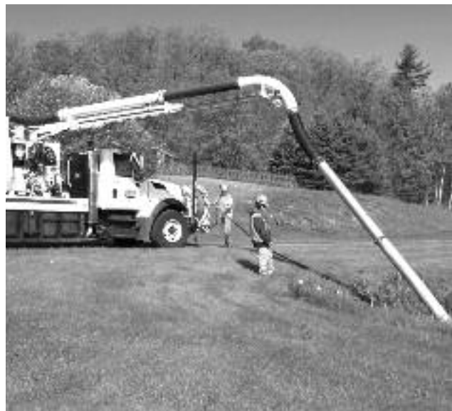
Vector truck cleaning out a stormwater pipe.
