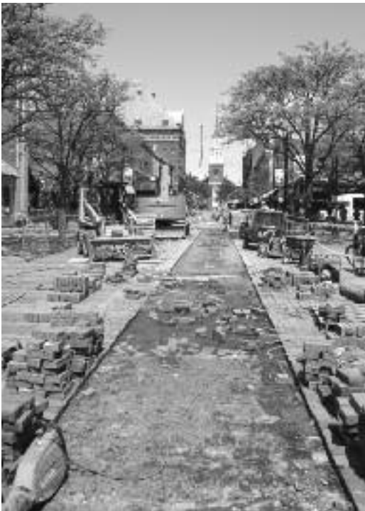
Church Street electrical and lighting project construction, summer 2012
