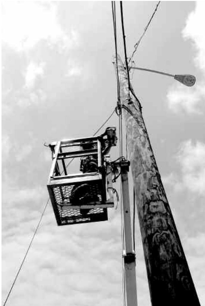
Worker installing a BT Line
