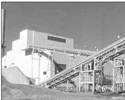
BED's McNeil Generating station
