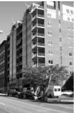
Westlake Condominiums, Battery Street
