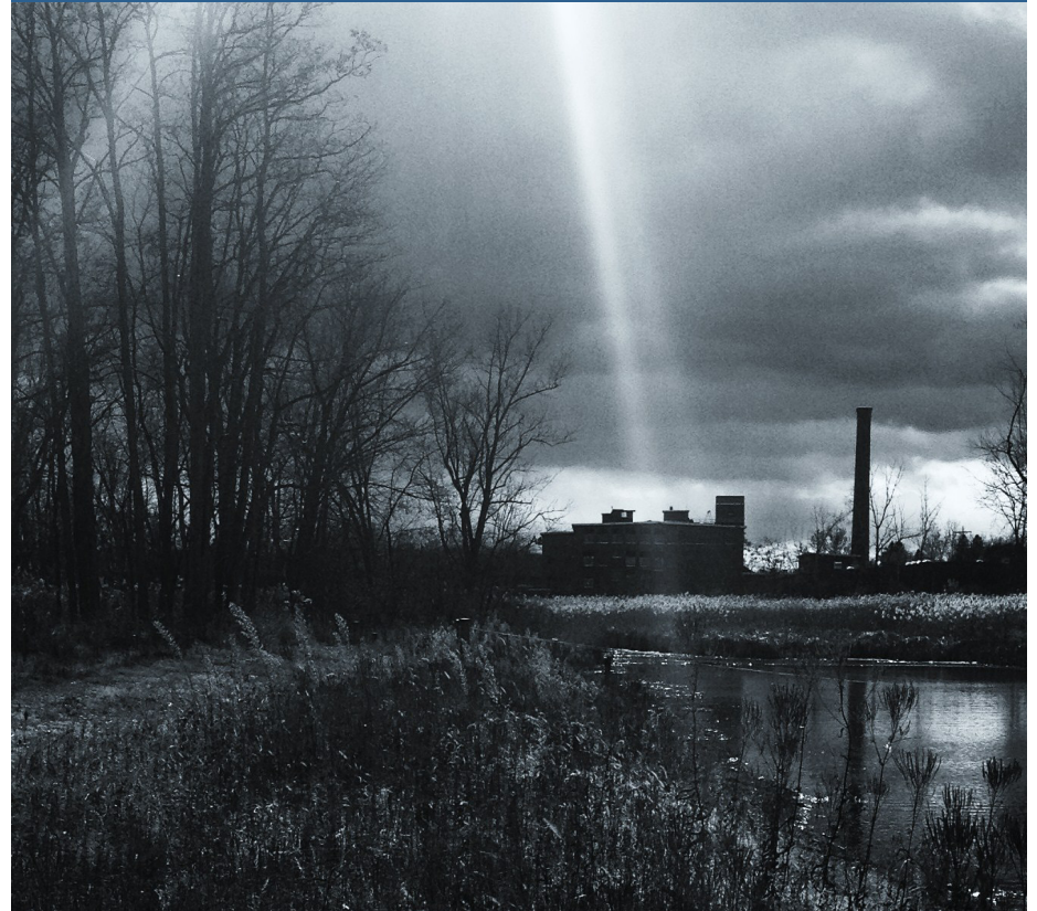
The Barge Canal Superfund Site has immense potential to once again become a productive part of the city's landscape—it blends nature and industry, history and ecology, beauty and grit. PHOTO CREDIT: DONNA WATERS
