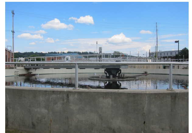
Waste water treatment facility
