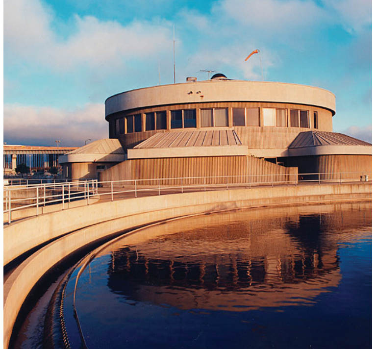
Settling tanks, big basins that hold wastewater, remove pollutants by collecting materials that naturally fall to the bottom and skimming off those that float to the top.
